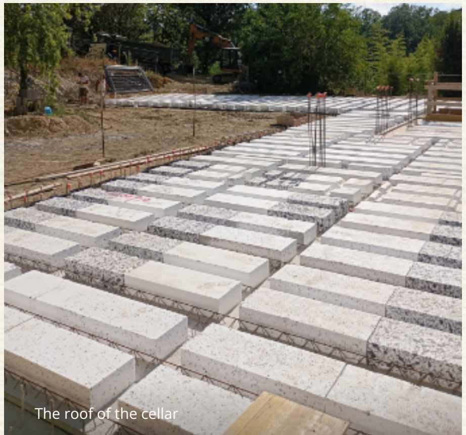
Placing the walls
