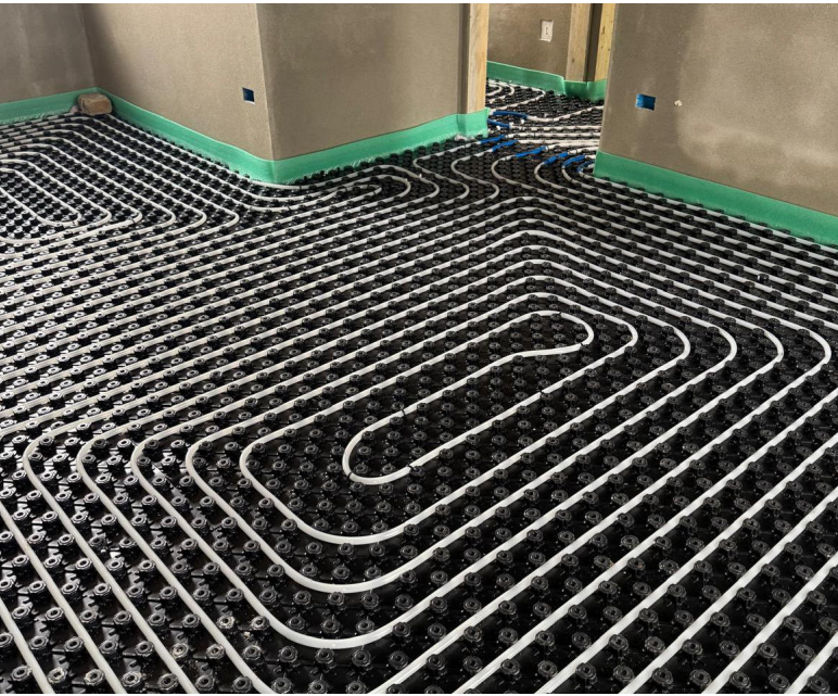
Placing floor heating
