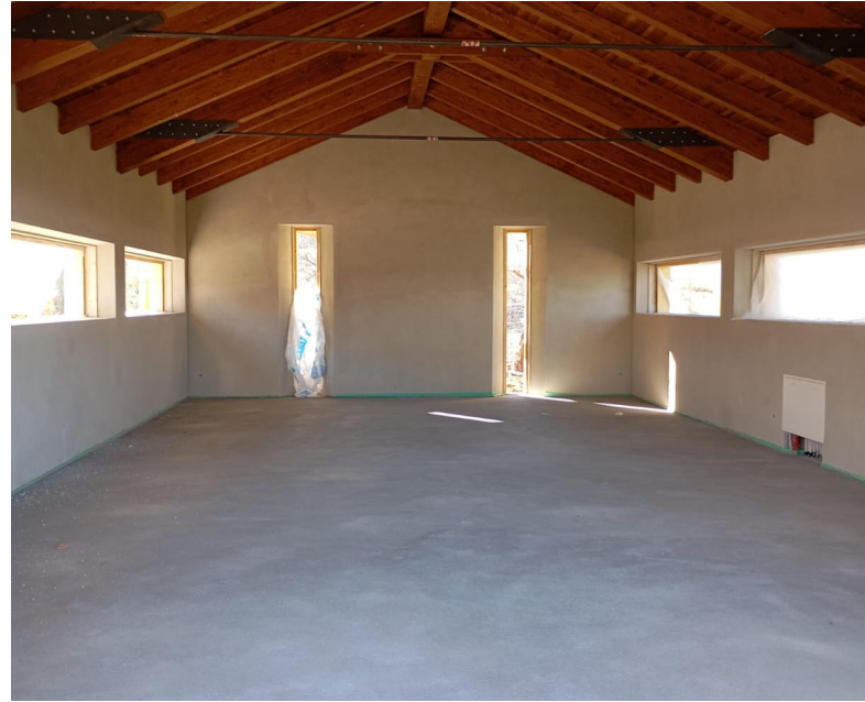
Pouring concrete floor
