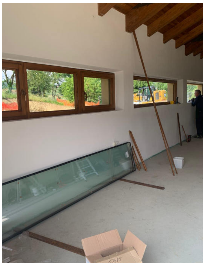
Placing doors and windows
