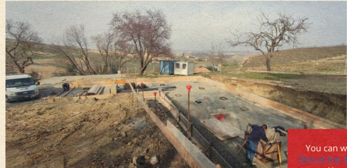
The foundation of the apartments
