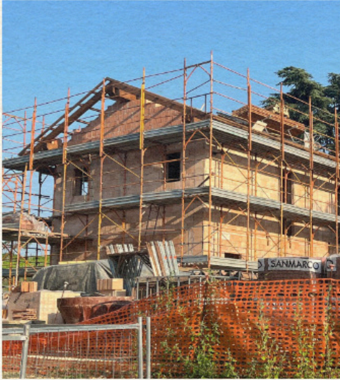
July: Building the roof
