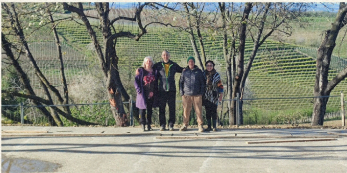
April: the foundation of the Dojo is ready
