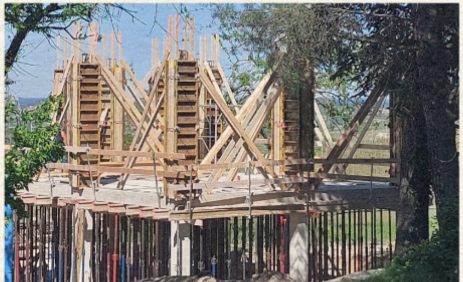
June: Starting the second floor
