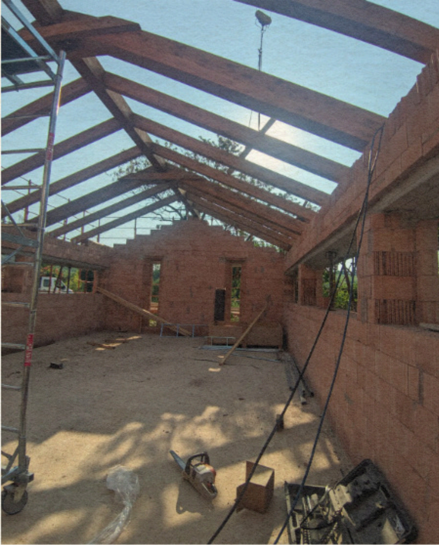
June: The construction of the roof
