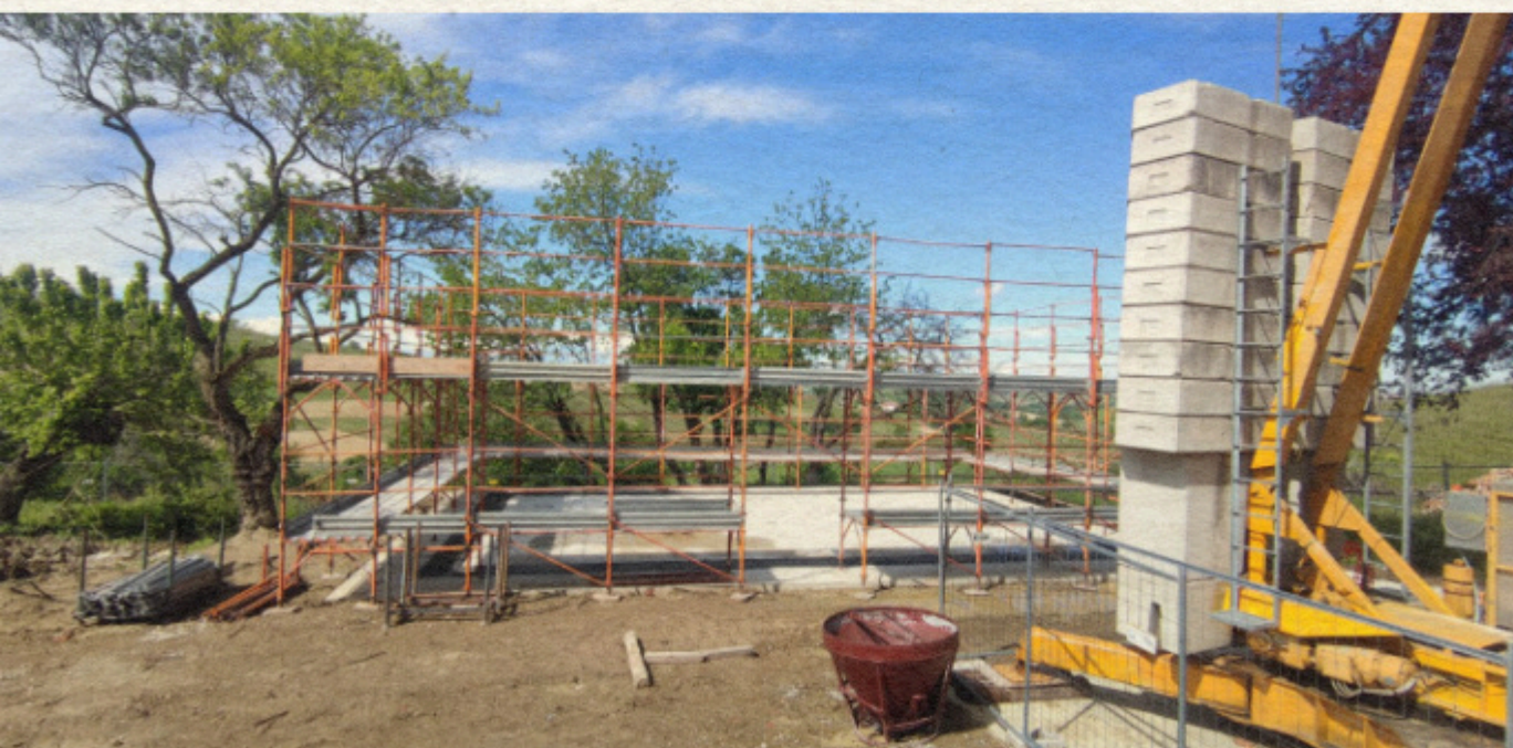
May: the walls are being erected
