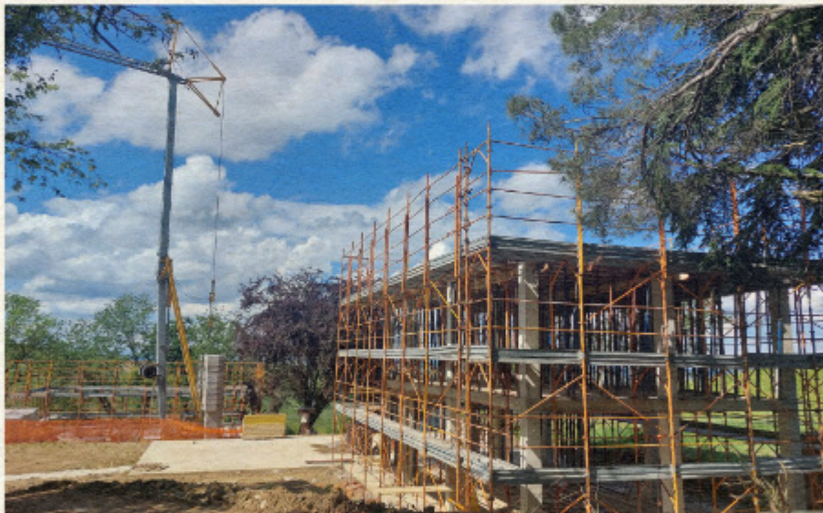
May: Constructing the walls
